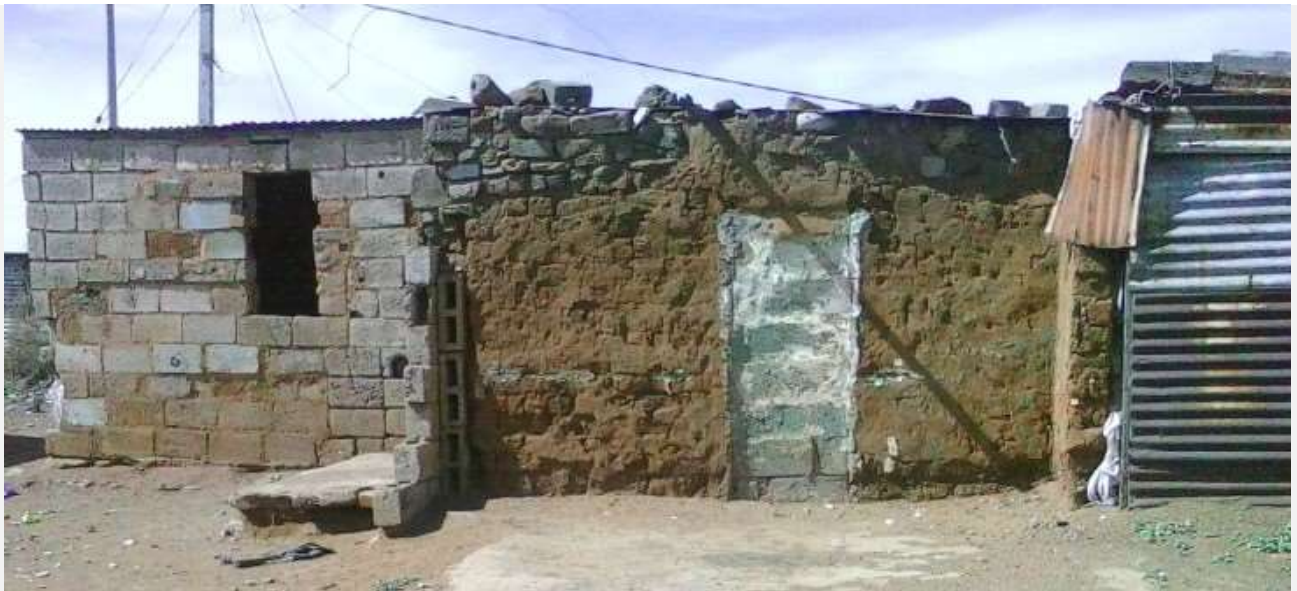
Illustration 3-11: An example of the structurally unsound houses in Evaton
